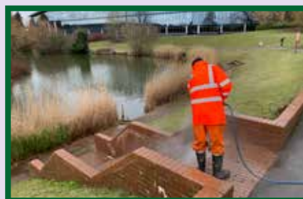
> Brickwork cleansing
